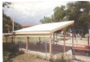
The completed daycare shelter.
